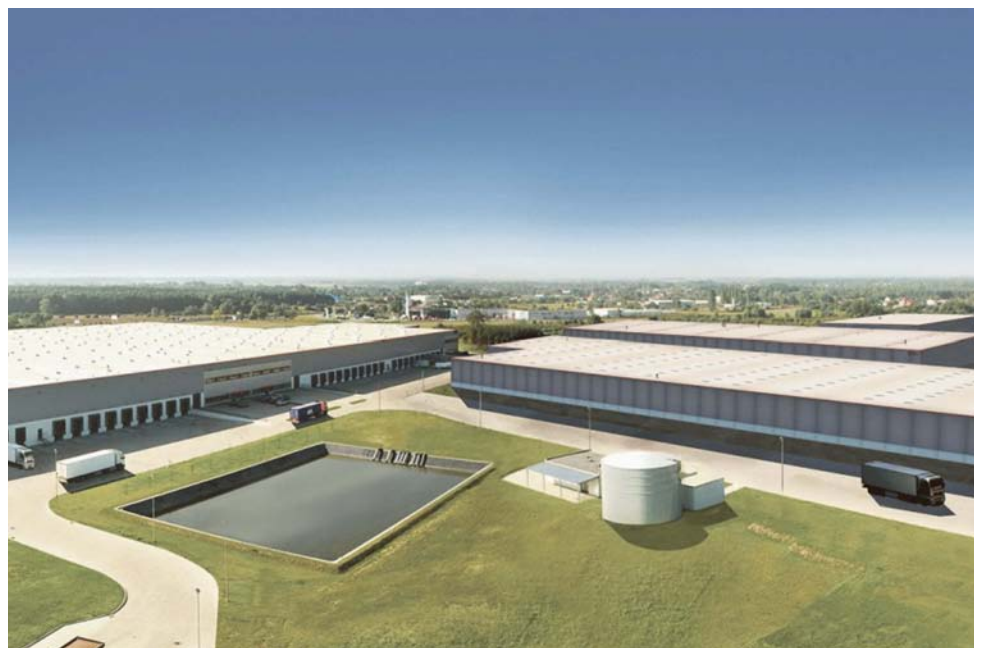
Segro Logistics Park Warszawa
