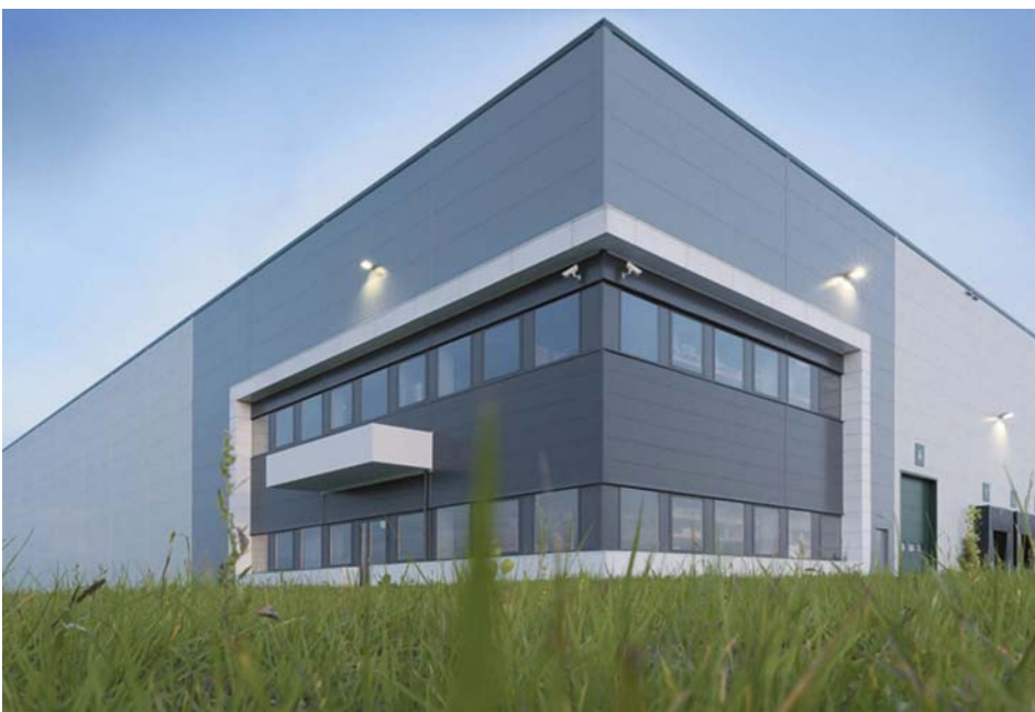
Prologis Park Wrocław
